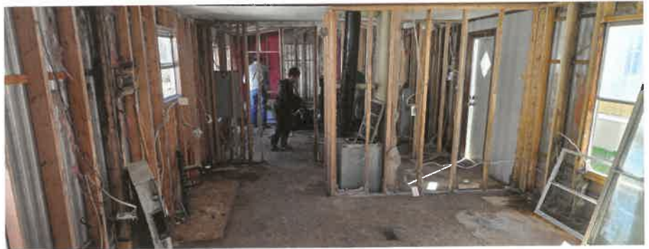
When they were finished, the homes had been gutted and were ready for the next phase of the process to begin.
